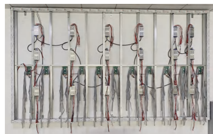
01 Install the frame and the power supply
